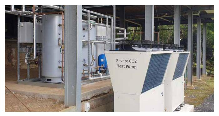
**Aged Care Facility, Beaconsfield VIC** 2 x 76kW Revere<sup>®</sup> CO<sub>2</sub> Air to Water Heat Pumps 2 x Thermex Stainless Steel Twin Coil Tanks 1 x Thermex Buffer Tank This customised hot water heating solution services both the domestic hot water and hydronic heating at this 90 room Beaconsfield Aged Care Facility.
